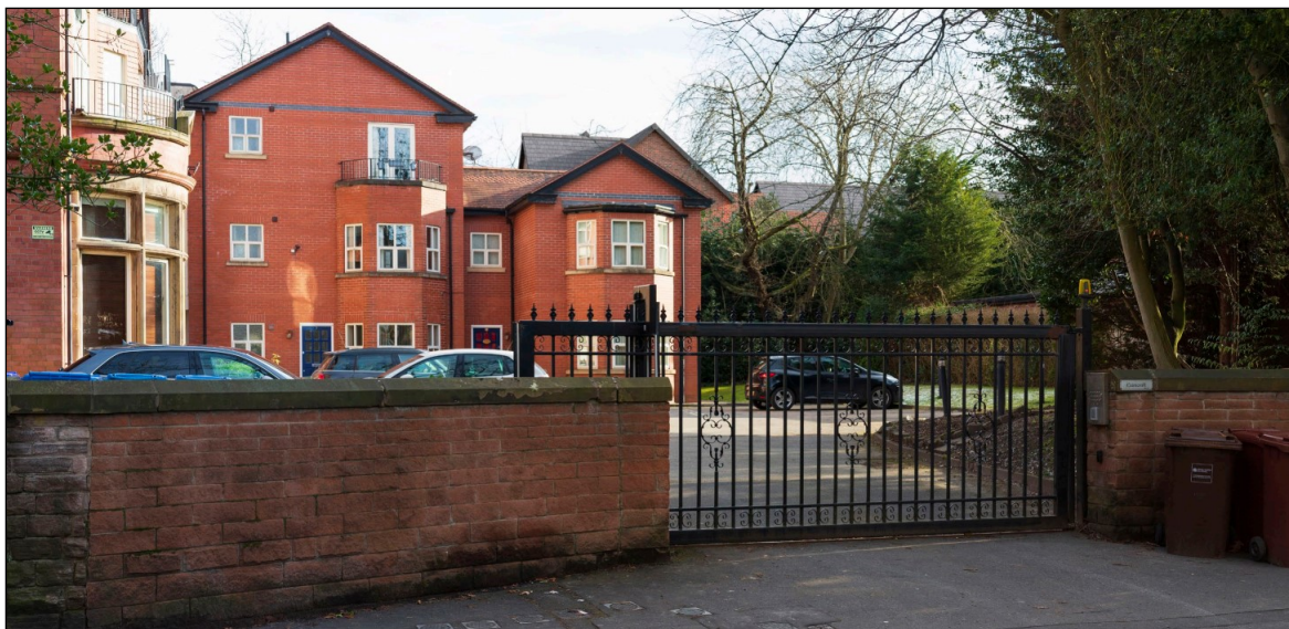
View from Holme Road of Cairncroft building with the building for the current application beyond
