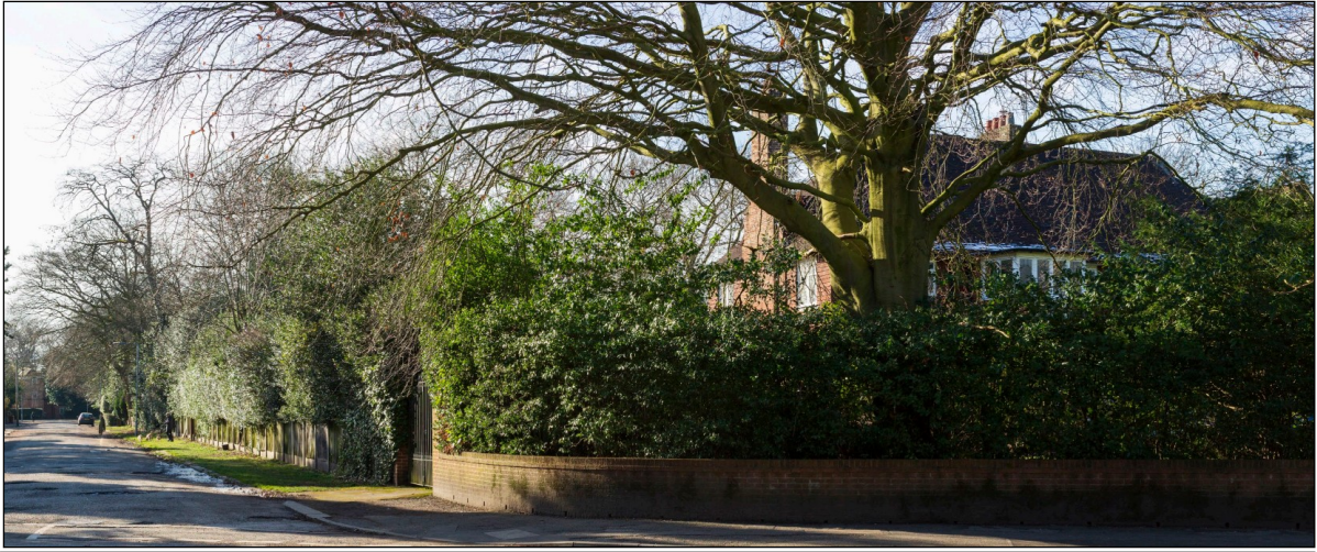
View of existing building from Spath Road/Lancaster Road junction
