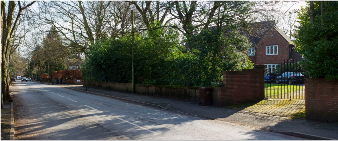
View of existing building from Spath Road
